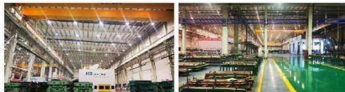
XCMG Factory Renovation Project, China
