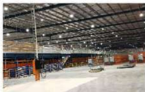
Toyota Motor Warehouse, Sydney
